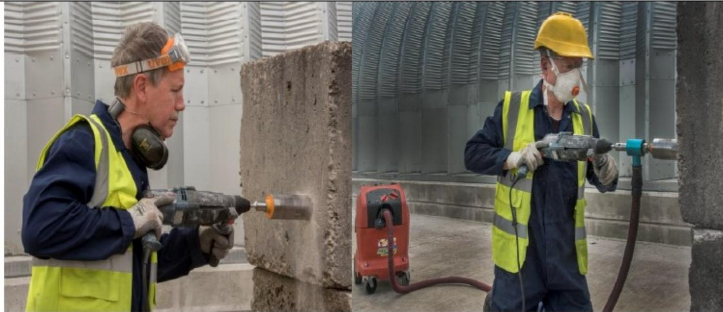
**Poor Practice** – Using hand-held corer with no extraction or RPE (HSE, GB)
