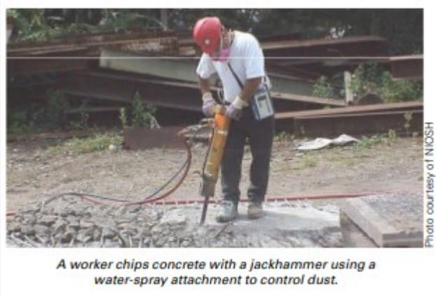
A worker chips concrete with a jackhammer using a water-spray attachment to control dust.
