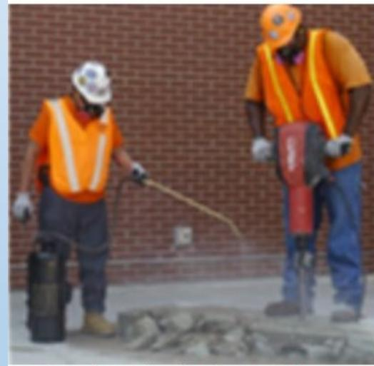
One worker applies water using a portable sprayer to suppress dust while the other jackhammers.
